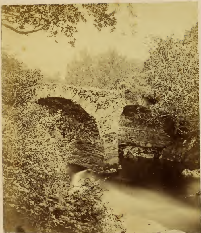
OLD WEIR BRIDGE.
